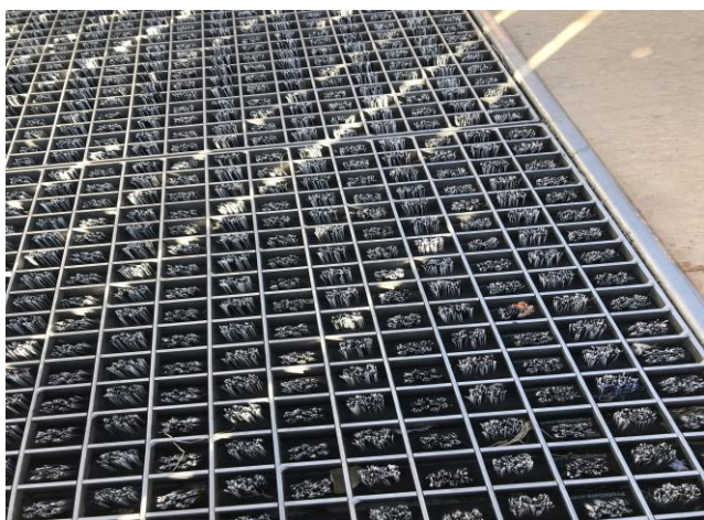
Photo 6: Containment strategy example 2: Pedestrian gate mats that capture the infill
