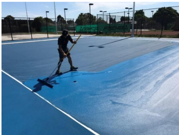
Photo 30: Application of Acrylic System
