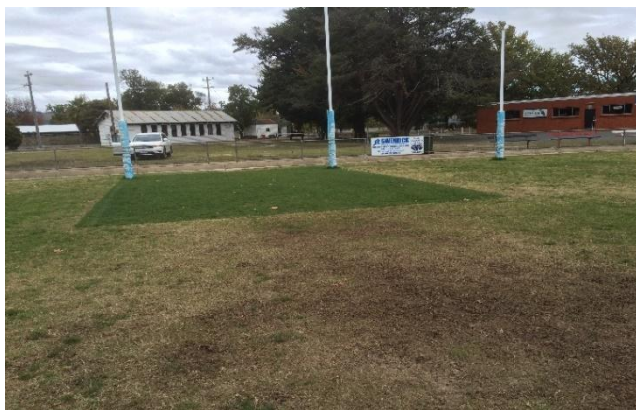
Photo 6: High Wear Area with Hybrid Surface in Goal Mouth (Source: HG Sports Turf)
