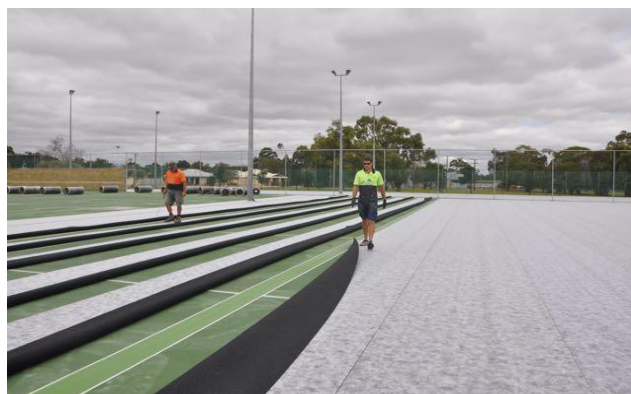
Photo 31: Installation of Prefabricated Mat System
