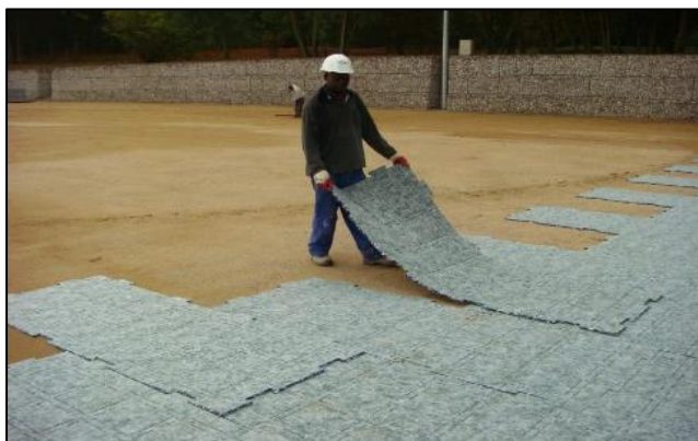
Photo 27: Prefabricated Shockpad Being Laid (Source: Team Sports)
