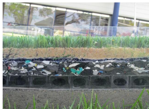
Photo 34: Example of Horizontal Drainage Cell Under Shockpad (Source: Wayne Stuart - City of Swan, WA)
