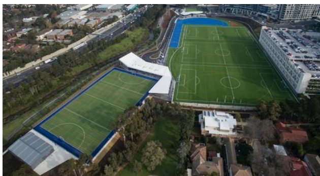
Photo 47: Multi-Sports Field at St Kevin's College, Toorak (Source: Tuff Group)
