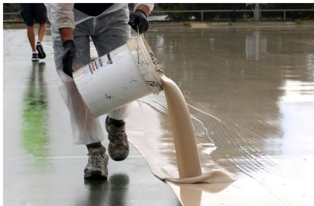
Photo 32: Application of Gel System
