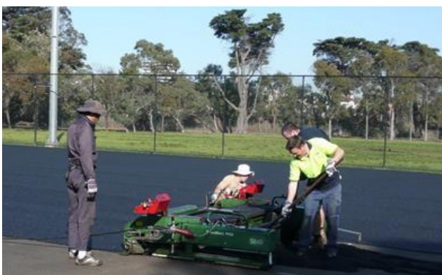
Photo 28: Insitu Shockpad Being Laid (Source: Polytan)
