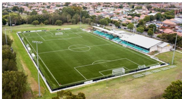
Photo 33: Bicentennial Park (NSW), which was Built Over a Closed Tip Site with Gas Capture Built into the Field
